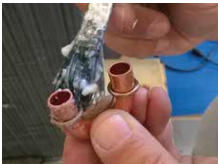
1. Flux is applied to the "U"-shaped returns
