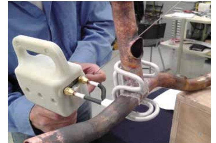
2. UBraze is positioned at the joint.
