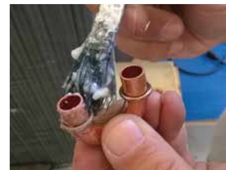
1. Flux is applied to the "U"-shaped returns
